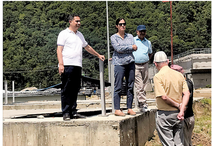
■ PID's Project Director Tires Prasad Khatri, ADB's Urban Development Specialist Vivian Castro-Wooldridge and PID's Consultant Engineer Dhruva Regmi inspecting Melamchi project infrastructure, at Sundarjial.
